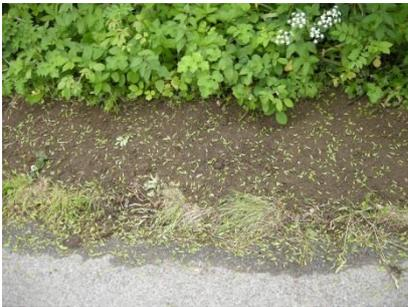
We are experimenting with how we restore the verge on Wood Lane where it has been damaged by heavy lorries associated with building work passing parked vehicles. To try to avoid any new topsoil being washed down the lane, we are placing a sod from higher up the bank at the road edge and then backfilling the verge with topsoil. We hope this proves more effective than previous repairs.
